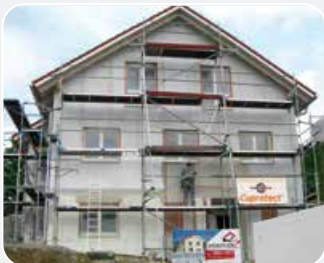
Exterior shielding embedded in ETICS
