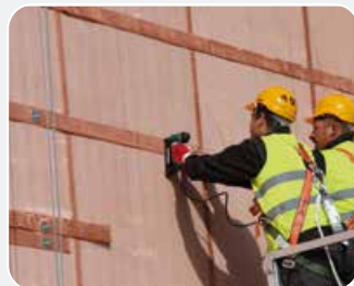
Exterior shielding in a dry construction system
