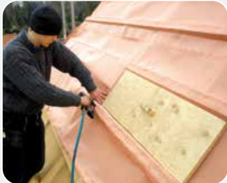
Top roof shielding
