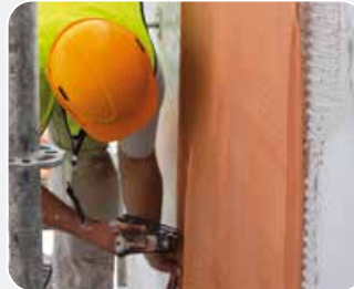
Exterior shielding embedded in plaster
