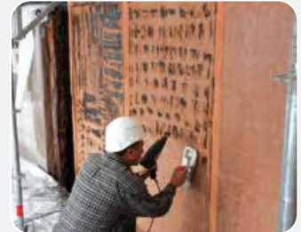
Exterior shielding embedded in hot bitumen
