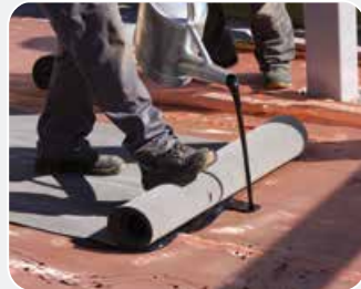
Flat roof shielding with hot bitumen
