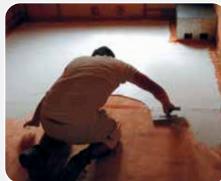
Floor shielding embedded in cement plaster
